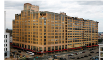
Equinix PH1 IBX data center exterior
